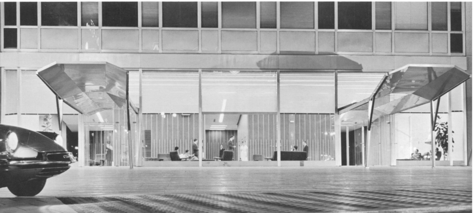
96. Main entrance canopies
