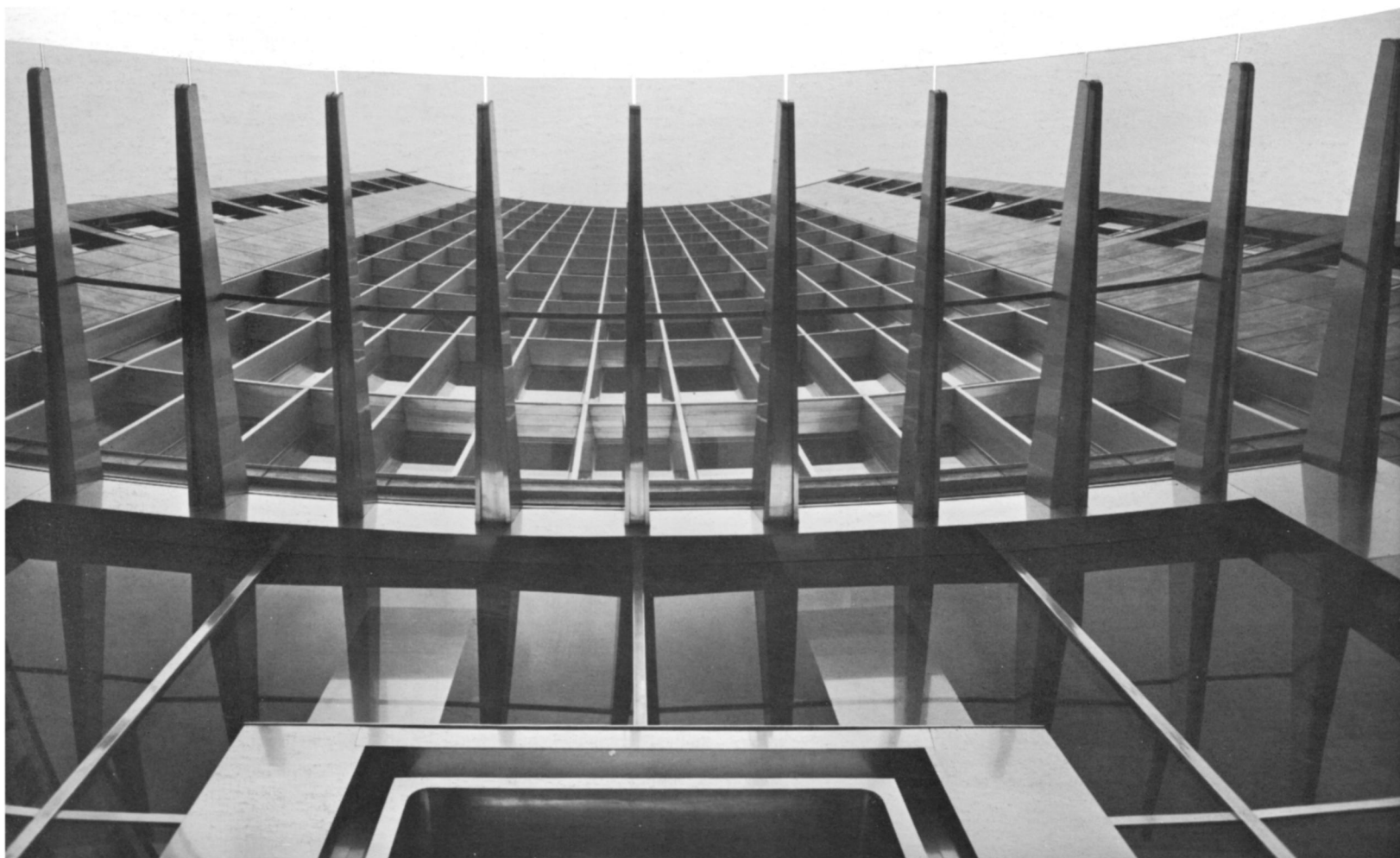
56. Main entrance canopy
